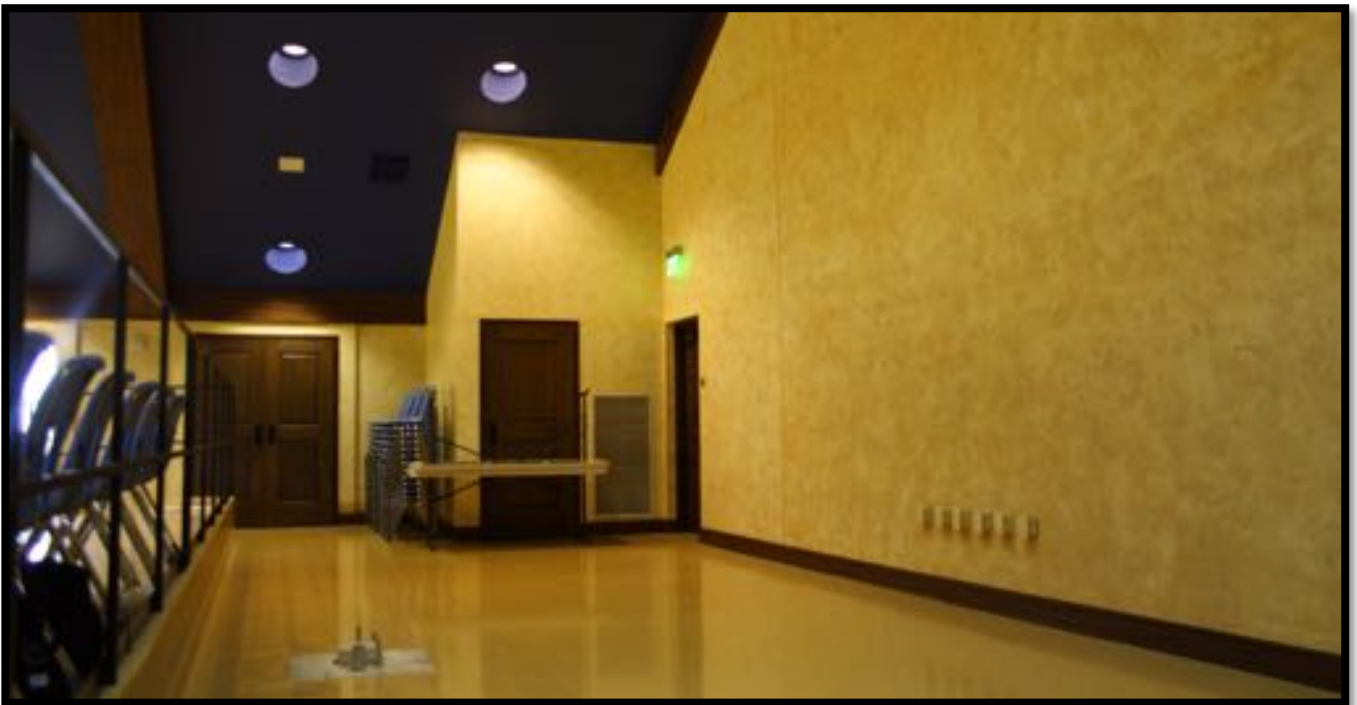
Space behind the choir risers was reserved for the eventuality of the pipe organ. During church construction, the infrastructure needed for the organ was incorporated. Note the electric boxes (to the right) on the back wall and the ductwork (lower left) in the floor. The ductwork supplies wind and power to the Rail Division, and connectivity for the Console in front of the choir risers. Additionally, the back wall was made of sealed masonry for its reflective properties.
